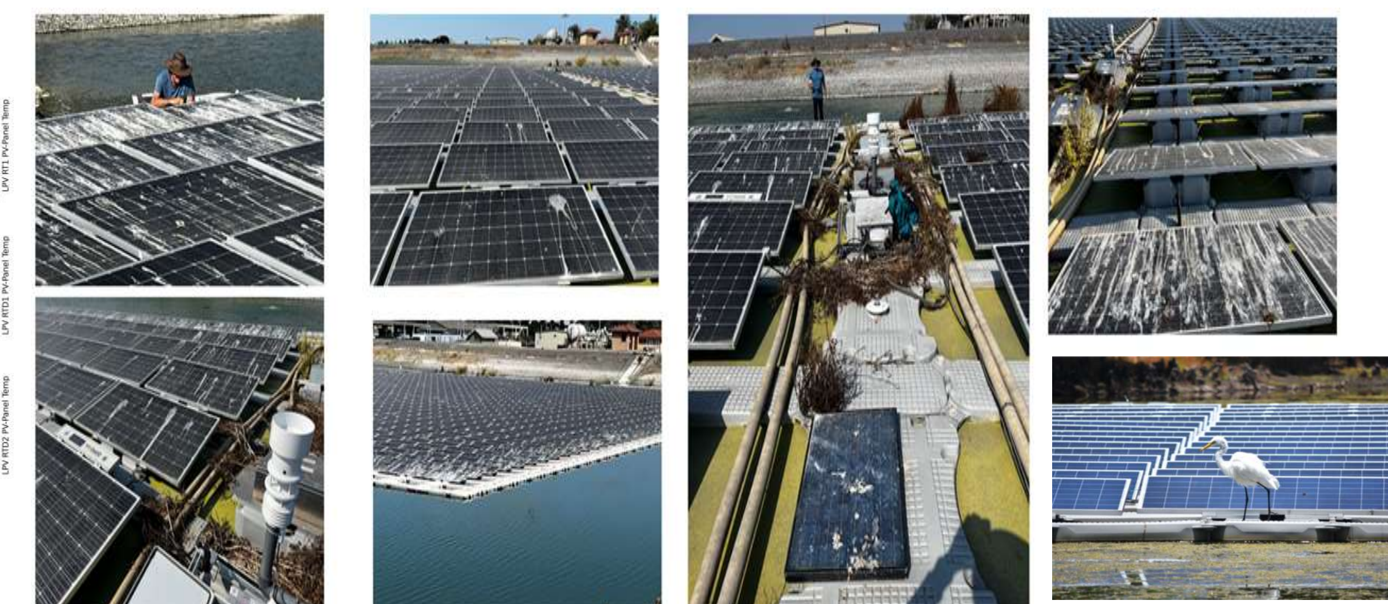
First six pictures: Bird droppings on a FPV located on a water treatment facility at Windsor, CA (Pic courtesy: Donard Metzger, Dave Chasar, FSEC, UCF); Seventh picture with bird: Great Egret utilizing the FPV platforms at a FPV, Orlando, FL. (Pic courtesy: UC Davis)
